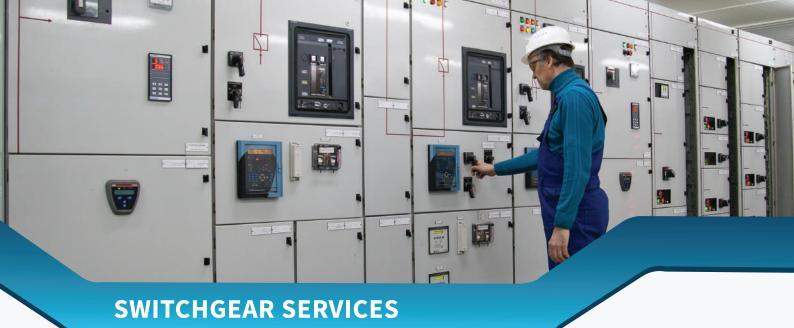
Switchgear is electrical equipment that is used to regulate, control and switching power supply and other devices in an electrical power system. It is a combination of electrical equipment like electrical meters, disconnect switches and fuses or circuit breakers.
